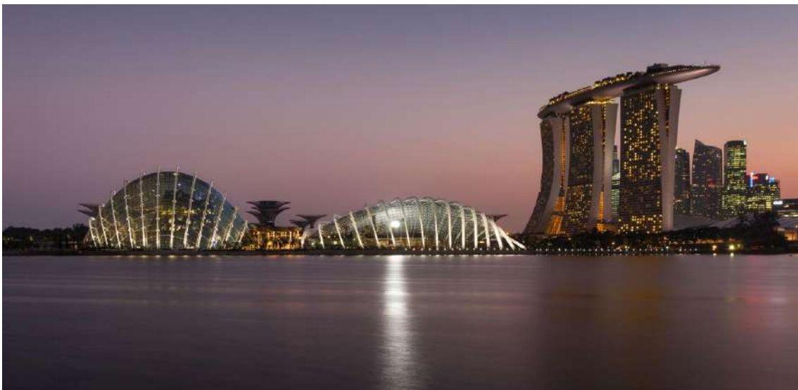
Figura 64 Invernaderos de Gardens By the Bay
