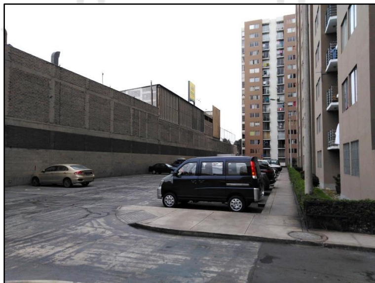
Figura 4.28 Condominio Alto Colonial – Supermercado Metro
