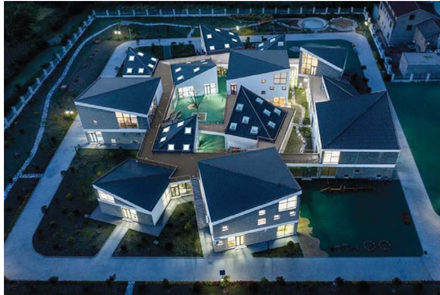
Figura 5-34 Jiangsu Beisha Kindergarten
