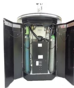
The 'Dry Side'
